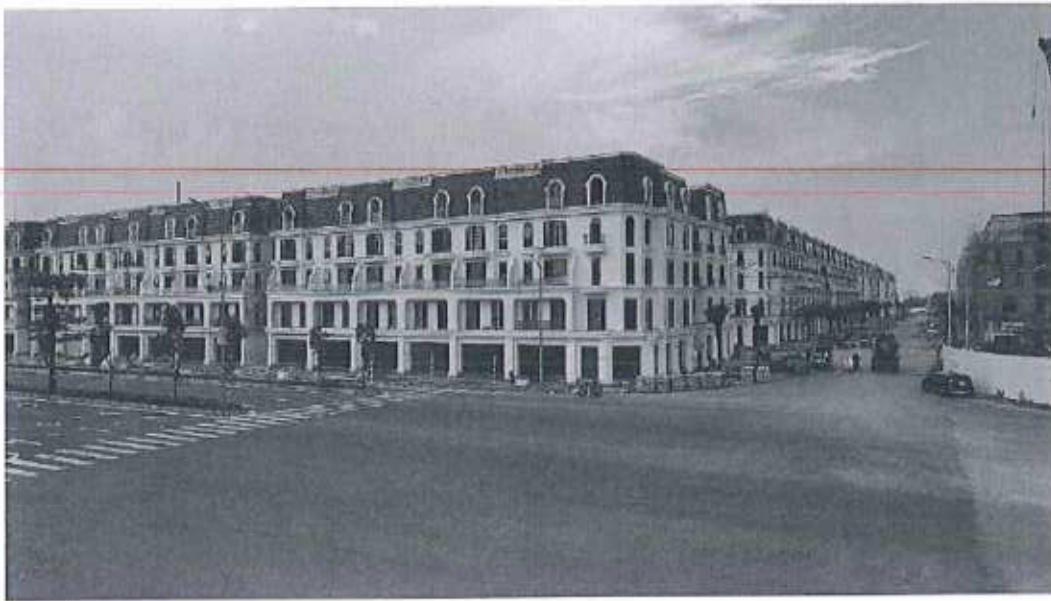
A corner of the project has been completed as of 07/2026
