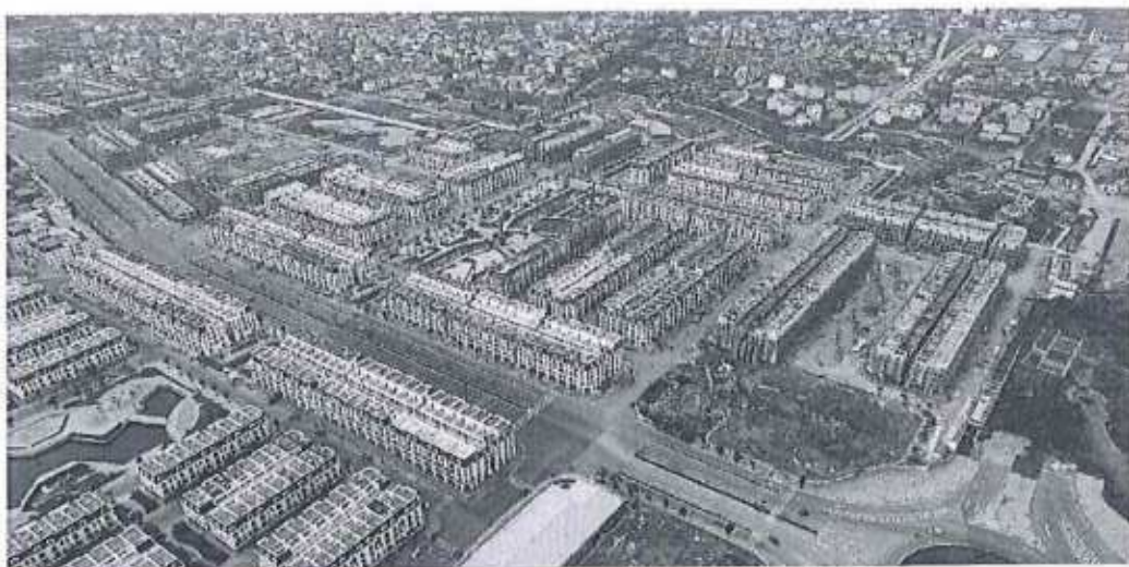
Overview of the project under construction is completing a number of subdivisions
